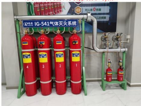
The IG-541 Inert Gas Fire Suppression System is a highly effective and environmentally friendly solution for fire prevention and protection. It utilizes inert gases to quickly and effectively suppress fires, making it a safe and reliable choice for a wide range of applications.
