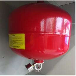
The hanging gas fire extinguishing device can be customized according to the volume size, type of fire extinguishing agent, and starting method. It is suitable for protecting areas such as power distribution rooms, transformer rooms, instrument equipment rooms, small oil depots, computer rooms, software libraries, communication rooms, archives and cultural relics reference rooms.
